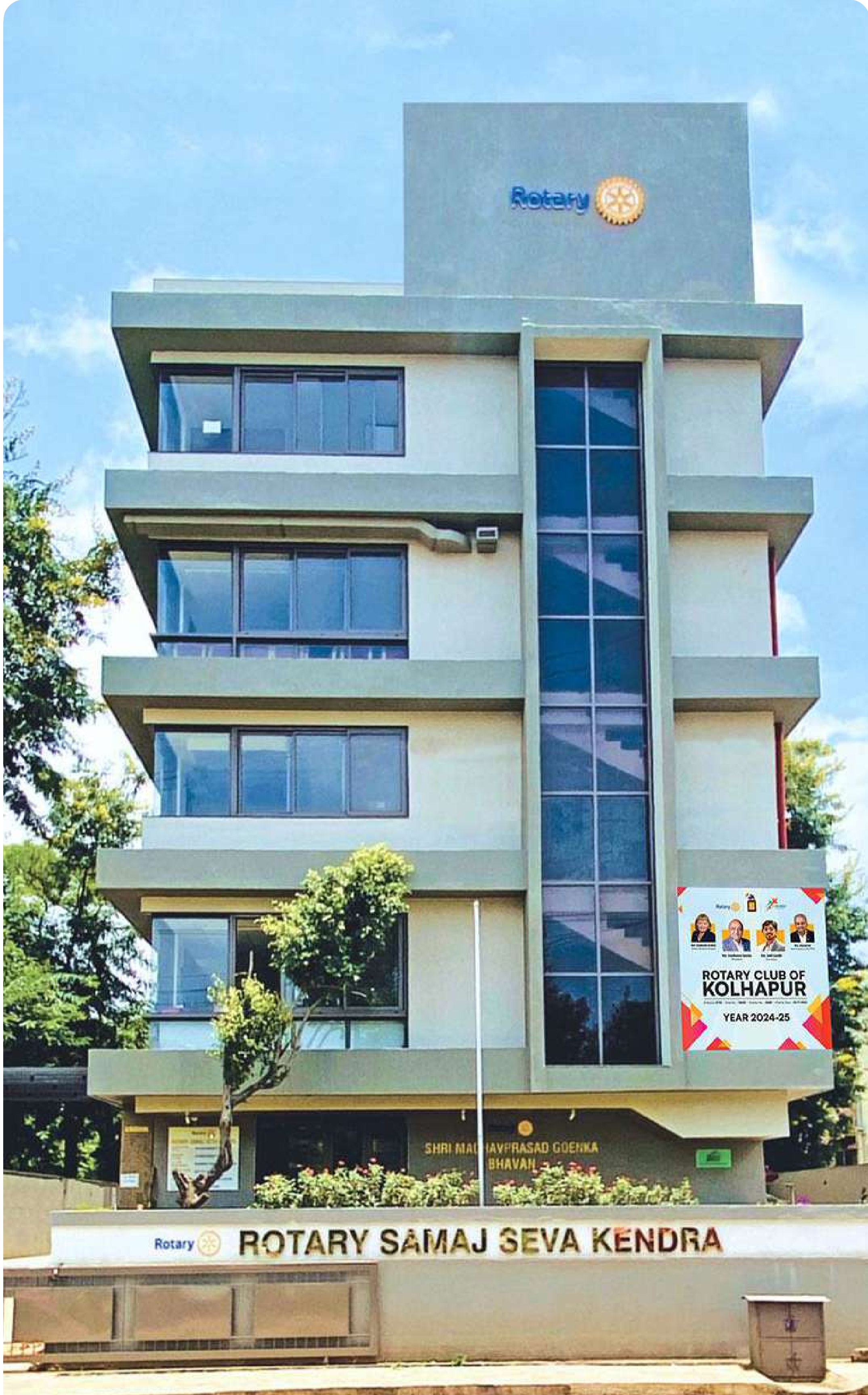
ROTARY CLUB OF KOLHAPUR'S ROTARY SAMAJ SEVA KENDRA BUILDING
